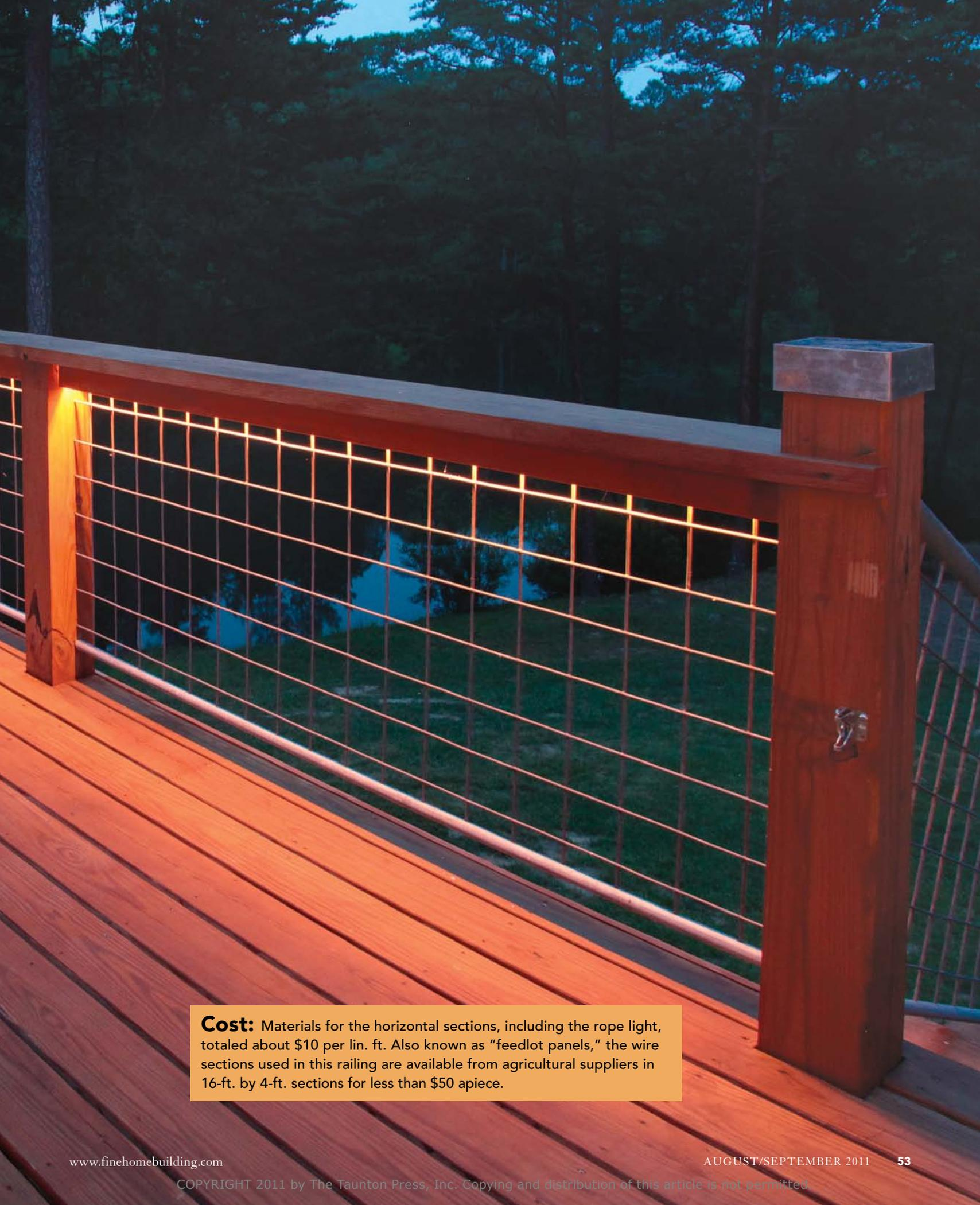
**Cost:** Materials for the horizontal sections, including the rope light, totaled about \$10 per lin. ft. Also known as “feedlot panels,” the wire sections used in this railing are available from agricultural suppliers in 16-ft. by 4-ft. sections for less than \$50 apiece.
