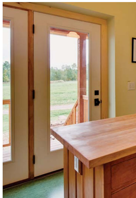
Outie doors need room to swing. Typical French doors have hinges on the jamb and can open only approximately 105° before hitting the inner part of the double-stud wall. If you don’t want to set the doors in line with the interior, use center-hinge doors.
