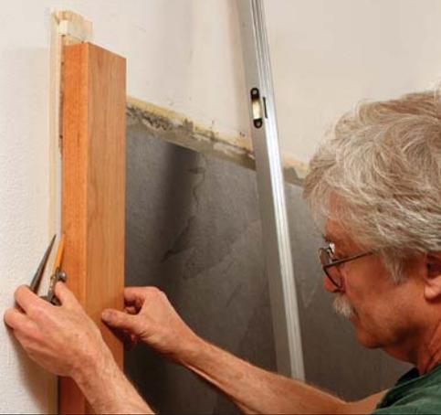
**The right setup.** After positioning the leg side-to-side, shim it plumb to the wall. Set the compass points to the widest gap, then draw scribe lines down both sides of the leg.
