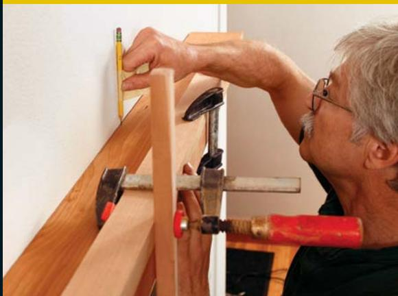
**Scribing with a crutch.** Instead of trying to hold the shelf in place while scribing, clamp a block to the shelf, then clamp to the block a long stick that reaches the floor.
