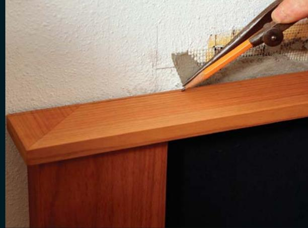
**Adjust the reveal.** To compensate for the uneven plaster, position the parting strip on the legs and use the compass to mark the amount to be scribed. The result should be an equal reveal over the legs on both sides.
