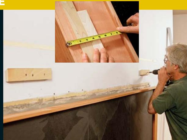
**Attach the wall cleats temporarily.** After measuring from the top of the shelf to the underside of the cleat (inset), transfer the cleat measurements to the wall. Use only one screw to attach each cleat so that it will be easy to adjust the cleat's position.
