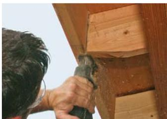
**Pull it in.** When the subfascia is too far out, cut back the rafter tails with a reciprocating saw.
