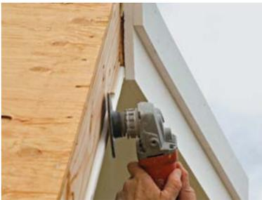
**Bevel the edge for a better fit.** Where the subsfascia can't be adjusted, use a right-angle grinder to remove material on the top edge of the soffit so that the fascia will install plumb and tight.
