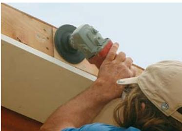
**Level the field.** The grinder comes in handy where adjoining lengths of subsfascia don't align.
