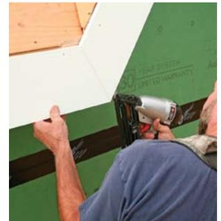
**One nail helps.** After finding the correct angle, cut and glue the fascia pieces, making sure they stay even with the plane of the roof sheathing. A 16-ga. nail provides insurance.
