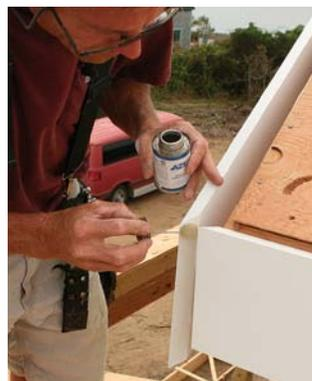
**Rake meets eave.** Miter and glue the rake's plumb cut, then mark and trim the bottom edge flush with the eave.
