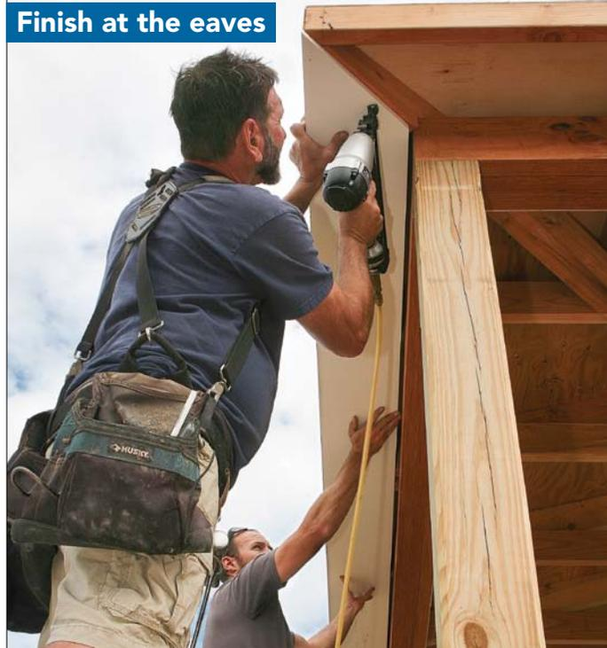
**Begin at the corner.** Start at one end of the soffit with a miter, keeping the outside edge flush to the subfascia.
