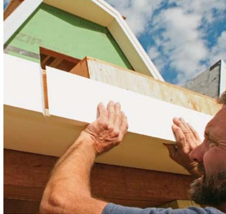
**Scarfs stay put.** At 45°, scarf joints offer more gluing surface than a butt joint. To keep a scarf from moving during installation, put a fastener at least a foot away from the joint, then glue and fasten the joint.
