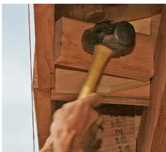
**Push it out.** Before the soffits are attached, use stringlines to check the straightness of longer runs of subfascia. Here, slightly longer blocking is hammered into place to push out the subfascia.
