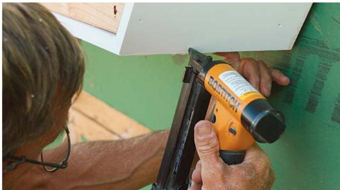
**Straighten as you go.** With the outside edge exposed, it's easy to straighten a wayward soffit with a well-placed shim.
