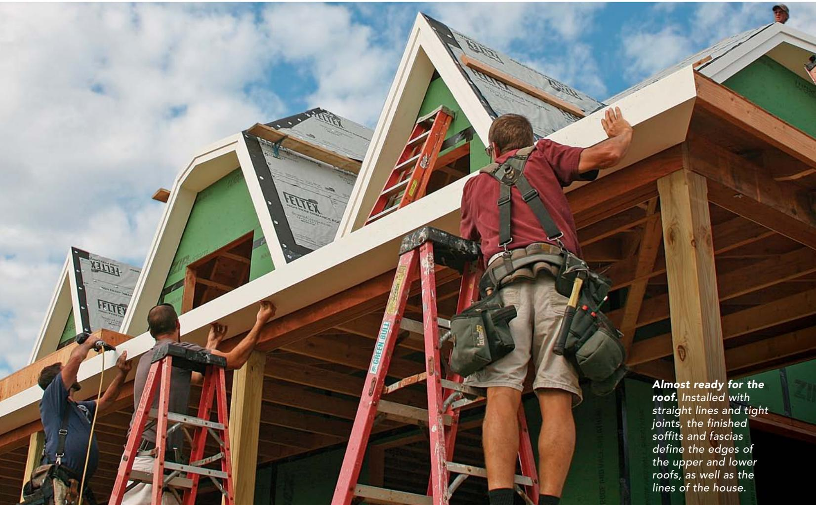
**Almost ready for the roof.** Installed with straight lines and tight joints, the finished soffits and fascias define the edges of the upper and lower roofs, as well as the lines of the house.
