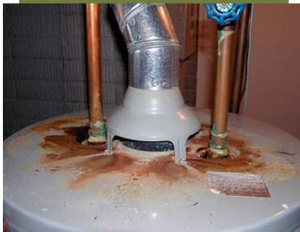
Clothes dryers, bath fans, and range hoods exhaust air from a house. If makeup air isn't supplied with a duct, it will leak in through cracks. Even worse, makeup air will be backdrafted through combustion appliances, which can cause carbon-monoxide poisoning. Using sealed-combustion appliances and makeup-air units for large range hoods gets around this problem.
