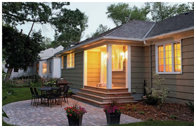
A new connection. Stepping back the addition at the dining room made space for a covered entry, which brings the backyard patio that much closer.
