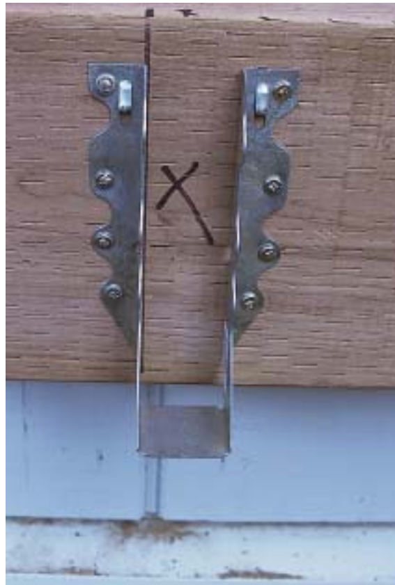
Hanger installed and ready for joist.
