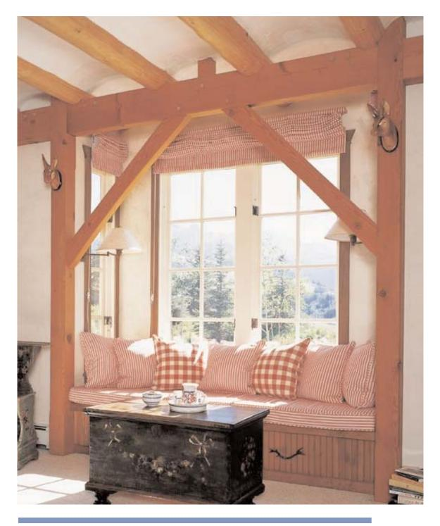
Timbers anchor and frame an extended bay, which is this bedroom's natural light and ventilation source. It's also an inviting window seat for reading, soaking in a little sunlight, or just enjoying the view.
