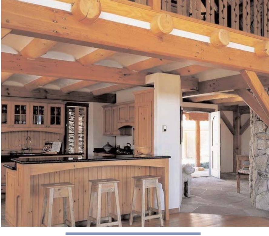
The Southwest design influence is evident in the extended log joists, the arched cavities between them, the rounded corners, the geometric pattern on the balusters, and the rustic post and capital detail on the porch. Timberframing is an elemental and adaptable building system. It doesn't dictate design style.
