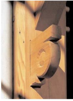
An oak spline, connecting to a beam on the opposite side, is extended to add strength to the joint. Its carved end is both decorative and structural.
