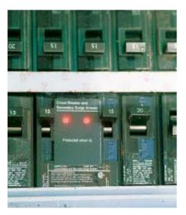
This two single-pole breaker module, made by Siemens, mounts in the main service panel like a standard breaker, but it also works as a surge arrester to protect the entire house. The lights indicate that the surgeprotection system is working.
