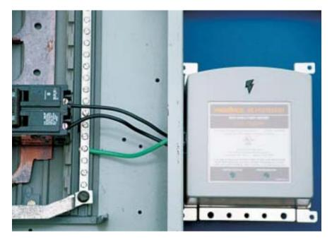
Although this Primax mounts outside the panel, it is encased in a metal box. The hardwired surge protector mounts on the side of the breaker panel and clips off surges coming in from the utility line. It receives power from a 30-amp doublepole breaker. Do not hide these within the walls.
