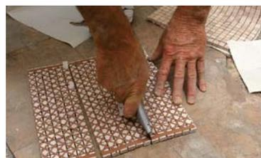
As long as you're not using glass tile, which requires a slightly different approach (visit [FineHomebuilding.com/extras](http://FineHomebuilding.com/extras)), you can install an accent band without changing your approach too much. Use a utility knife to cut sheets of mosaic tile into strips, set them into the thinset with firm pressure, and adjust individual tiles as needed to keep things even.
