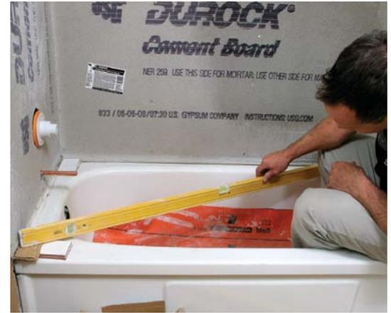
**Know your tub installation.** It would be nice if every tub installation were dead level, but that's rarely the case. Before you can begin the tile layout, lay a level across the top of each side of the tub. The bottom row of tiles can be cut to follow the contour of the tub or to account for high spots, so the goal here is to find the low point, which becomes the starting point for the rest of the layout.
