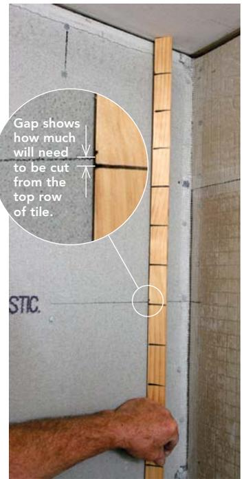
**Flip it for the ceiling.** Turned end for end and placed against the ceiling, the story pole indicates the amount that needs to be cut from the top row. Here, the cut will leave almost an entire tile, which is perfect.
