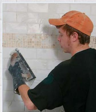
**Spread and scrape.** Use a margin trowel to load grout onto a rubber float, and then use the float to apply it to the wall. Spread the grout in broad, arcing strokes. Start with your arm extended, and pull the float toward your body. The first pass packs grout into the joints; the second pass scrapes away most of the excess.
