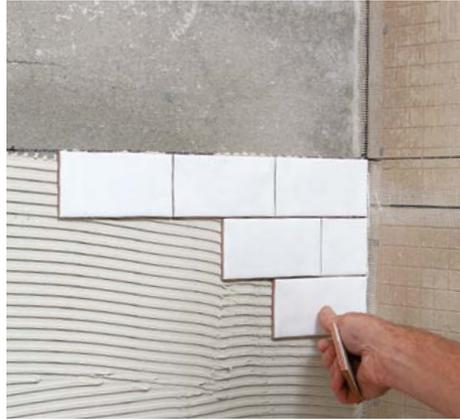
**The first tile establishes the pattern.** On this job, the story pole confirmed that a full row of uncut tiles could fit along the back wall, so the first row begins with a full tile, followed by a half-tile below it to establish the running bond pattern. If a full row of uncut tile won't fit, it's better to start in the center of the wall and have the same cut on each end.
