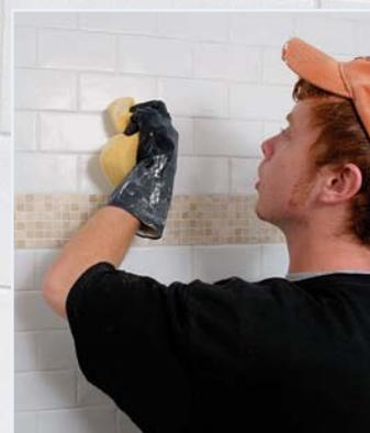
**Wipe away the haze.** Once the tile has been washed down and all excess grout removed, let everything dry for about 15 minutes, or until a light haze develops on the surface of the tile. Then use a clean cloth or quality paper towel to wipe the haze off the surface of the tile, buffing it to a finished shine.
