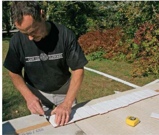
**A stick tells the story.** Cut a piece of wood for the vertical layout and another for the horizontal layout, each a bit shorter than the distance between tub and ceiling or wall and wall. Place the tiles one at a time, including a space for grout between each if the tile isn't self-spacing, and mark the layout on the stick.
