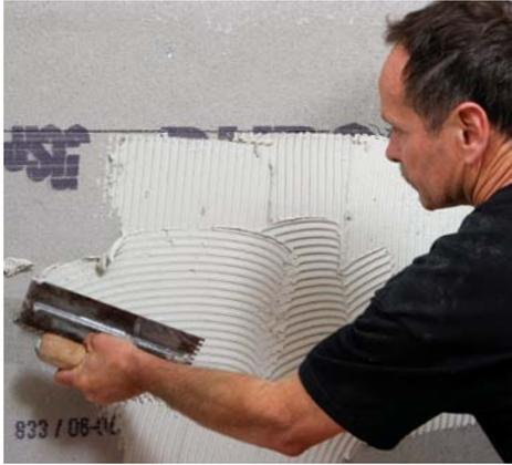
**An even spread.** Working from the benchmark line down, start with the lower part of the back wall, spreading the thinset cement with a 1/4-in. square-notched trowel. Use a sag-resistant latex-modified thinset such as Laticrete 255 for tub surrounds because it reduces the chance that tiles will slide out of position before the cement sets up.
