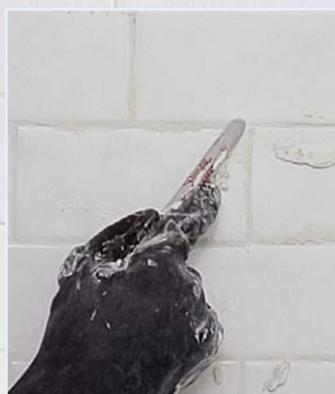
**Pack and tool the joints.** Once the grout has firmed up but before you wash down the tile, use the butt end of a Sharpie permanent marker as a grout stick to strike the grout joints. This packs in the grout tightly and makes the joint consistent.
