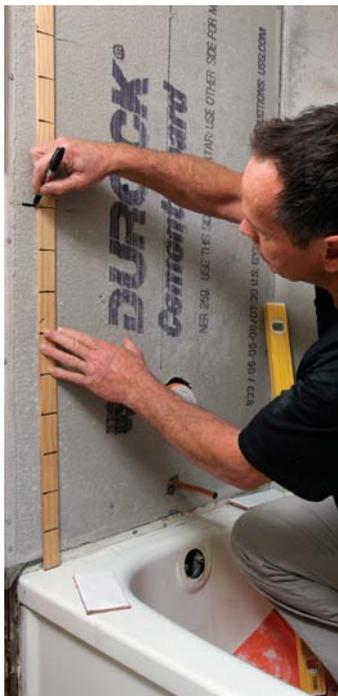
**Up from the bottom.** Set the end of the story pole on the tub's lowest spot, then draw a mark at least halfway up the wall that corresponds to the joints of your story-pole layout.
