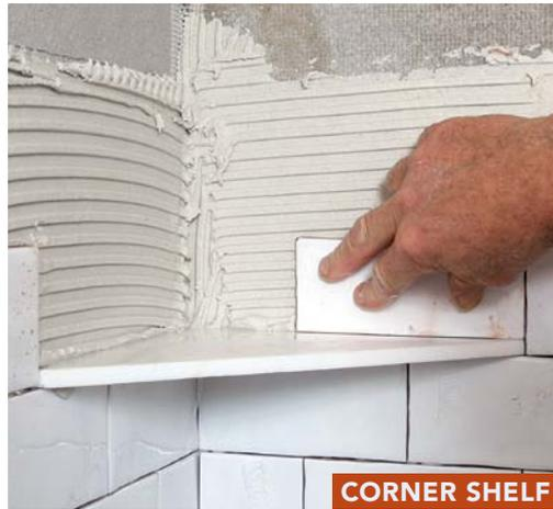
I typically make a corner shelf from a 12x12 stone tile. Here, I cut a piece of marble in half diagonally and then rounded over the edges with a rub brick. Installation is easy: Butter the back edge of the shelf with thinset and rest it atop a course of tiles. Trim the next course of wall tiles as needed. To keep water from pooling on the shelf, put a few temporary plastic wedge spacers under the shelf, all the way at the back of the corner, so that it sets up with a slight pitch.
