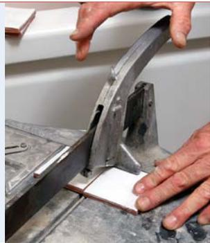
**Score and snap.** For all straight cuts, a basic snap cutter works quickly and makes a clean cut. Score across the top of the tile, then give the handle a quick bump with the palm of your hand to break the tile at the score line. If the cuts are difficult, small, or notched, a tile saw is a better choice.
