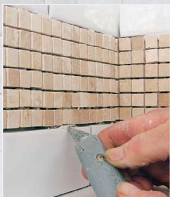
**PregROUT cleanup.** Before mixing up the grout, spend a few minutes looking over every joint in the tub surround. Even a day after it's been applied, the thinset is still fresh enough to be removed easily with a utility knife.
