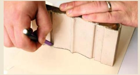
**Take a sample.** The most accurate method of copying a molding profile is to trace the profile's contour onto a piece of heavy paper. To minimize the hazards of working with materials that could be covered with lead paint, wear a respirator and gloves.
