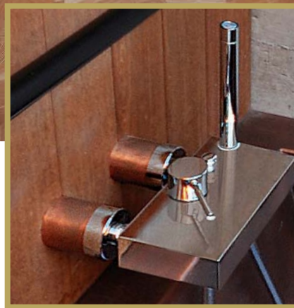
Squared off. Rectilinear shapes at different scales abound in the baths, from the end-grain Douglas-fir flooring to the Duravit Starck X toilets. Practical issues included the need to create custom copper sleeves to extend the pipes for the tub mixer (inset).
