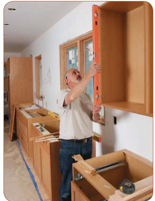
**Do your own work in order.** Countertops take a couple of weeks from measurement to installation. Start interior trim by installing the cabinets so that the countertop measurements can be taken, then continue on to the doors and trim.
