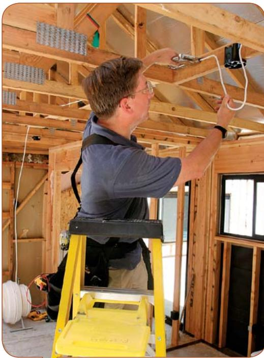
**Bring in mechanical trades in a specific order.** Ducts are the least flexible mechanicals, so they go in first, followed by the plumbing. Wires take up little space and can go almost anywhere, so schedule the electrician last.
