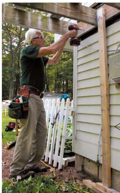
Once the deck frame was back in place, we added two more 2x8s to the outside rim board so it would be adequately sized as a beam (removing the dip in the original one in the process). We made sure the crown, or arch, in the new members faced upward to help counteract the downward bow in the existing rim joist. When finished with the reinforcement, we added support posts between the new footings and the beam.
