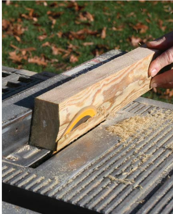
Peaking the railing. The top and bottom rails were each beveled at 10° to shed water. They were then sanded and the bottom edges rounded over.
