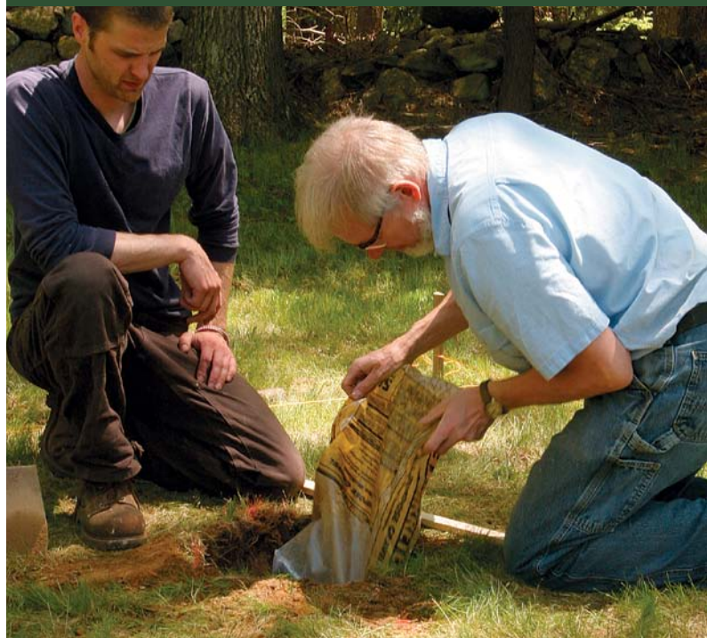
Dump in some gravel. Filling the bottom of the hole encourages drainage, which minimizes the chance of frost heave.
