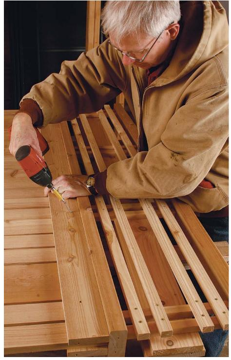
**Screw on the subrails.** Drive  $2^{1}/4$ -in. stainless-steel trim-head screws through the faces of the 1x4 and 1x6 subrails. Angling the screws matters here; not only does it tighten the subrails to the 2x4s, but it prevents the screws from running out the opposite face.
