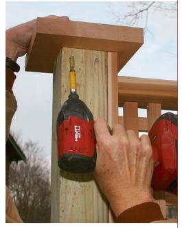
**Fasten the cap.** You can use pocket holes and screws to attach the cap to the post, or you can bed the cap in silicone caulk.
