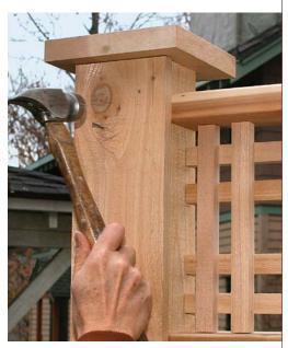
**Fasten the facing.** Attach the 1x cedar with stainless-steel 6d siding nails or stainless trim-head screws, which cost more but make it easier to remove the facing for repairs.
