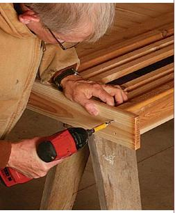
Attach the side pieces. These 1x4s will be the anchor point between the panels and the posts and will transfer the weight of the panel, as well as any side loads from wind, to the 4x4 posts. Attach them with a pair of  $2^{1}/_{4}$ -in. stainless-steel screws driven through each rail and subrail.
