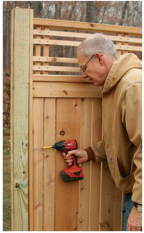
**Screw the panel to the post.** Drive four  $2^{1}/2$ -in. stainless-steel screws through both the front and back sides of the panel to attach it to the first post. Set the panel on blocks so that it's level, drop the second post in its hole, and fasten the panel to the second post. Holding the post plumb, fill the hole with gravel and concrete.
