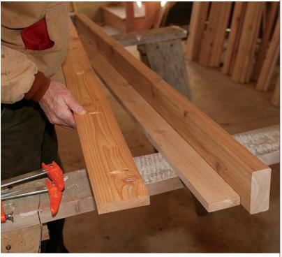
**Spacer creates an even reveal.** Place the 2x4 center rail on its edge atop sawhorses with a 1x spacer next to it. Align the ends of the subrail with the ends of the center rail.
