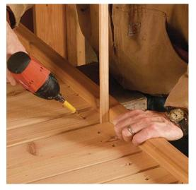
Angle the screws. With a narrow panel board spaced from its neighbor with the gauge stick, drive in a single 1<sup>1</sup>/4-in. screw (two screws for the wide boards). Angling the screws helps to drive the panel boards tight to the 2x4 rail.
