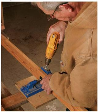
**A pocket-hole jig creates angled screw holes.** Clamp the jig (kregtool.com) onto the 1x4 or 1x6 subrail that will be on the fence's show side. A special bit with a collar drills perfectly angled, stopped screw holes in the subrail's hidden face.
