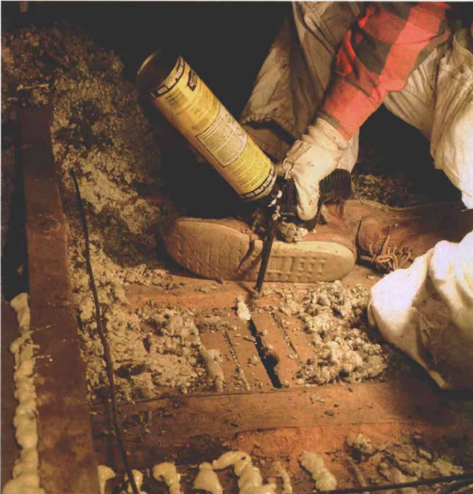
Smaller holes and cracks can be filled with caulk or foam. After attic insulation is pulled away, holes can be found and filled. Here the author fills cracks in a plaster-and-lath ceiling.
