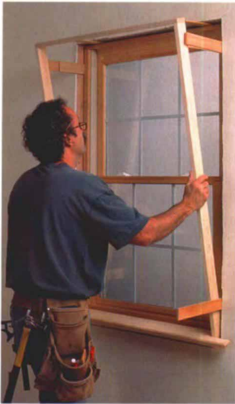
Installing the jamb extensions as a unit. After tapering the pieces individually, the author cuts them to their final length and assembles them into a unit with the stool.
