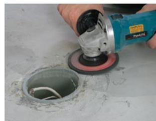
Flooring manufacturers specify that the slab not exceed  $\frac{3}{16}$  in. in flatness over a 10-ft. span. I always check the entire slab with a 10-ft.-long straightedge and mark any spots that are lower or higher. For the lower areas, I mix a batch of floor leveler and use the straightedge as a screed. It usually takes a couple of coats to level out a large area. Small high spots can be ground down with an angle grinder.
