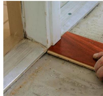
**Trim door casing before you start.** To make the installation easier, it's a good idea to cut door casing so that the flooring can slip beneath. Flooring contractors often use a jamb saw, but you can do the same job with a handsaw and a scrap of flooring as a guide (see p. 118).
