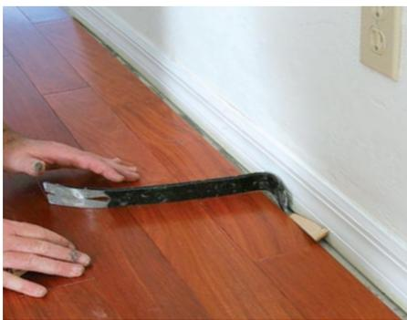
**Keeping the edges tight.** Cut from scrap, small wedges keep the flooring joints tight along the  $\frac{3}{8}$ -in. gap at the baseboard.
