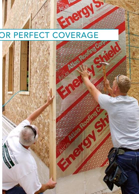
**Marking the panels in place is easier than measuring.** Around rough openings, it's just as quick and more accurate to lift the panels into place to mark them rather than take measurements. Mark the panel for the horizontal cuts, and measure the distance from the furring strip to the closest panel for the vertical cut. Use a T-square to draw cutlines, and cut through the panel in one pass with a **heavy-duty snap-blade knife** ([www.tajima-tool.com](http://www.tajima-tool.com)).
