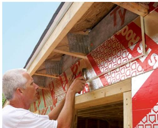
materials I typically use. When I decided to include rigid-foam insulation in wall assemblies, I had to consider how it would affect the entire wall system. For instance, the foil-faced polyisocyanurate used here is a vapor barrier, so I eliminated the interior vapor barrier of the original design.
