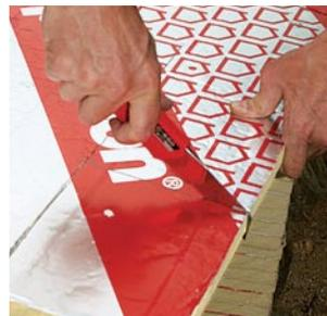
**Insulate between the rafters, but leave an air gap at the roof.** Cut small pieces of insulation to fit between the trusses (or rafters), making sure they stop at least  $1\frac{1}{2}$  in. shy of the underside of the roof sheathing. This gap keeps air flowing into the attic.
