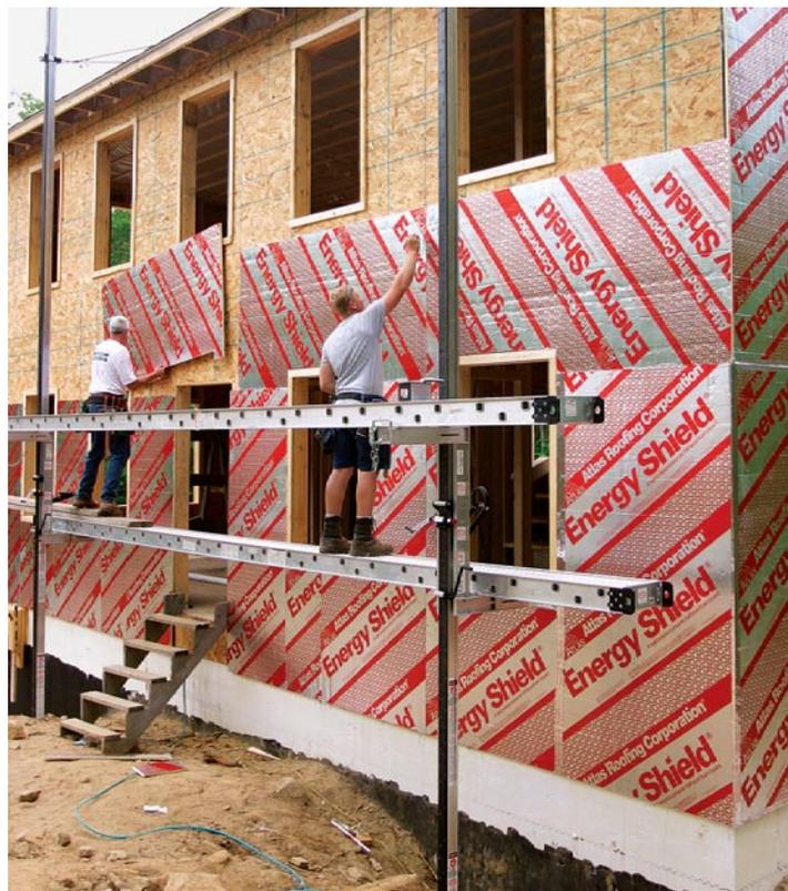
In a typical wood-frame house, about 25% of the wall area is composed of uninsulated wooden structural elements. Relatively speaking, wood is not a good insulator, and the thermal bridge it provides conducts heat from one side of the wall to the other.
