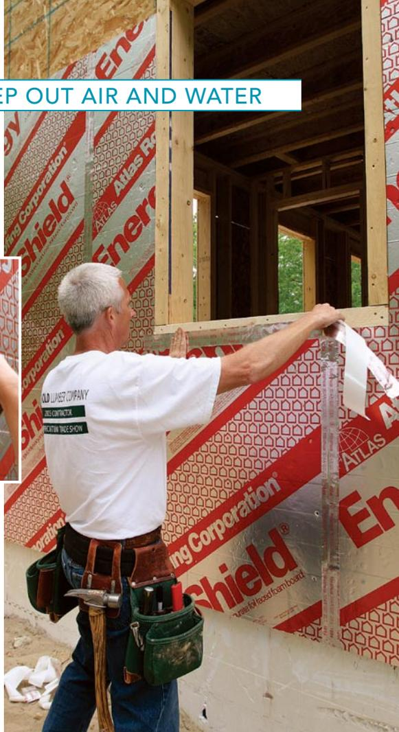
back and fasten the panels every 12 in. on center around the edges and 16 in. on center in the field. Manufacturers recommend fasteners with at least a ⅜-in. head, so I use aluminum roofing nails. Cap nailers also work well.
