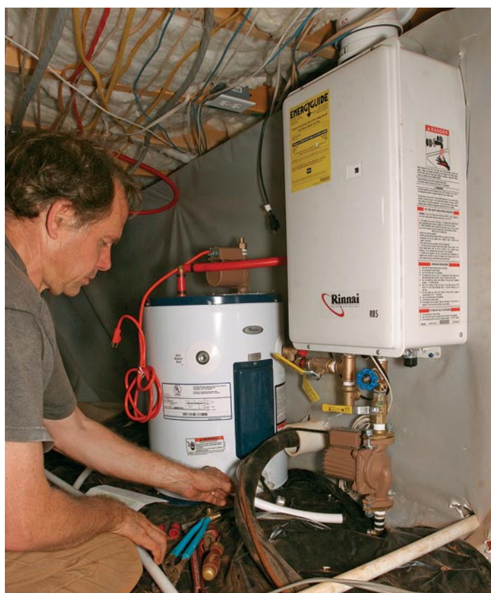
No floor space required. Because the water-heating system is so compact, it can fit comfortably in a crawlspace.
