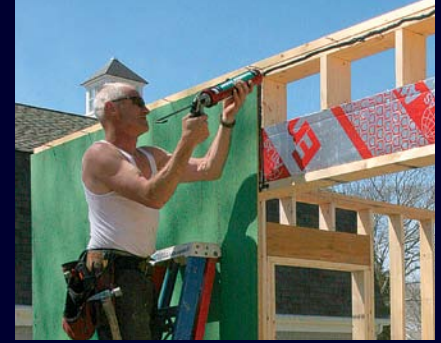
Sheathing air barrier. Panel sheathing makes an excellent air barrier. Seams should be sealed with long-lasting, high-stick tape, and holes should be plugged with foam or caulk. Acoustic sealant is sometimes used to seal gaps between the sheathing and the framing.
